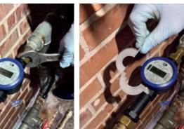
A technician from Tårnby Forsyning in the process of replacing a mechanical meter with a remotely read meter.
